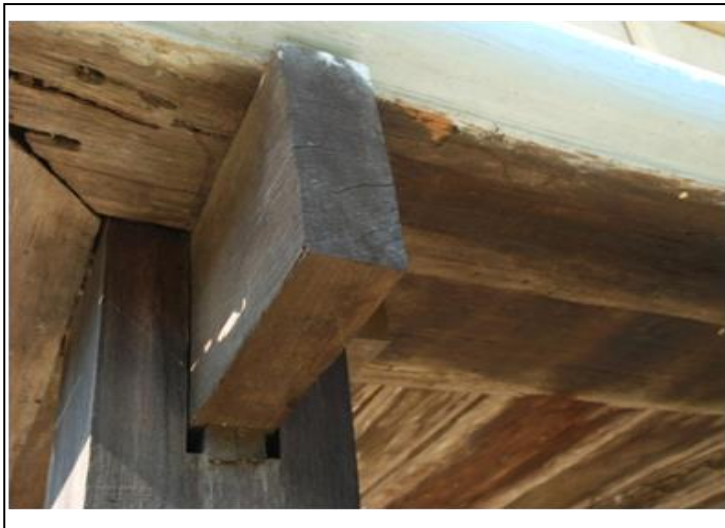
Figure 6: Floor joint of Kampung Tuan Mosque.
