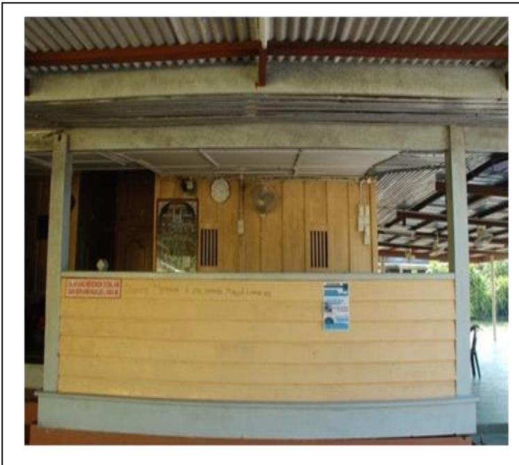
Figure 23: New veranda and asbestos ceiling finishes.
