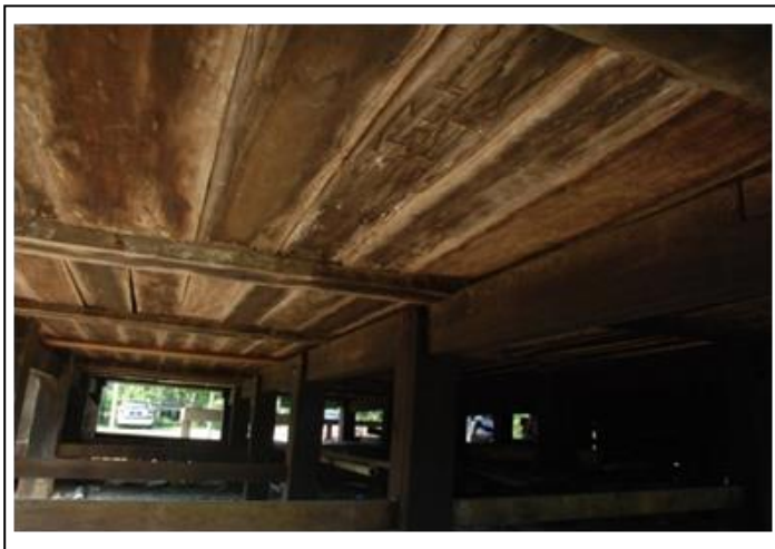
Figure 9: Removable timber floor panel of Kampung Tuan Mosque.
