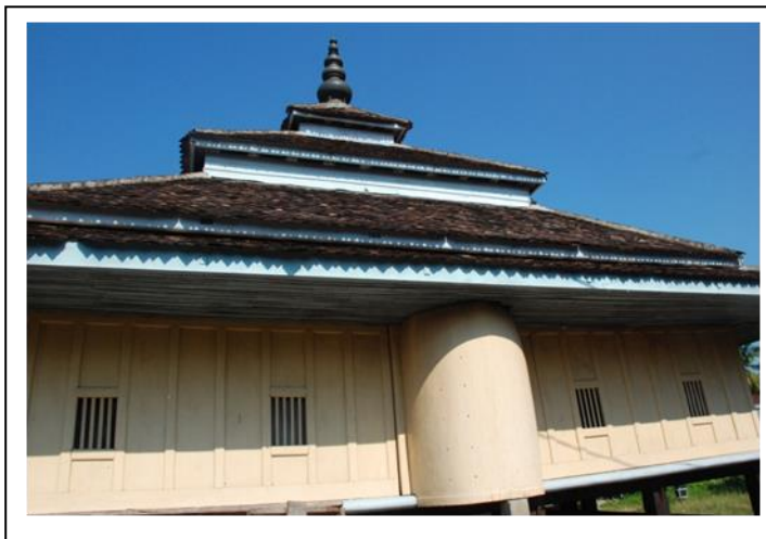
Figure 19: Mihrab wall and windows of the Kampung Tuan Mosque.
