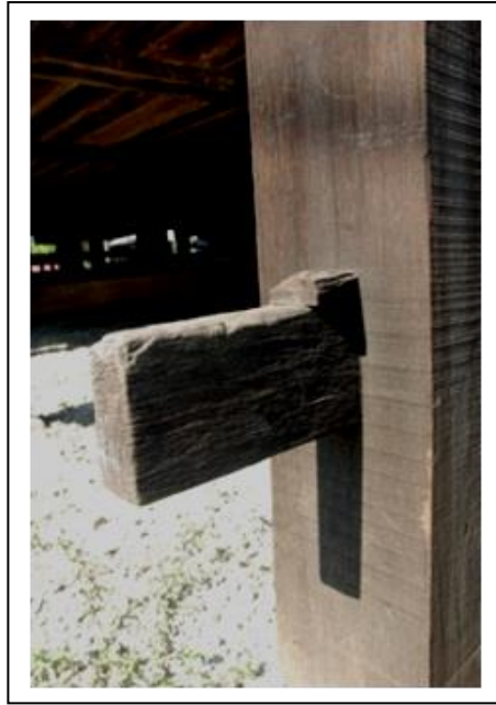
Figure 7: Column joint of Kampung Tuan Mosque.
