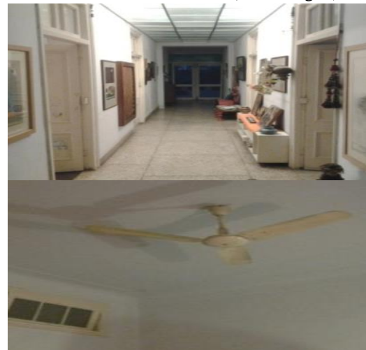
Fig. 7. Entrance Passageway of Traditional House (upper) and Traditional Ventilator (lower), Source: Author
