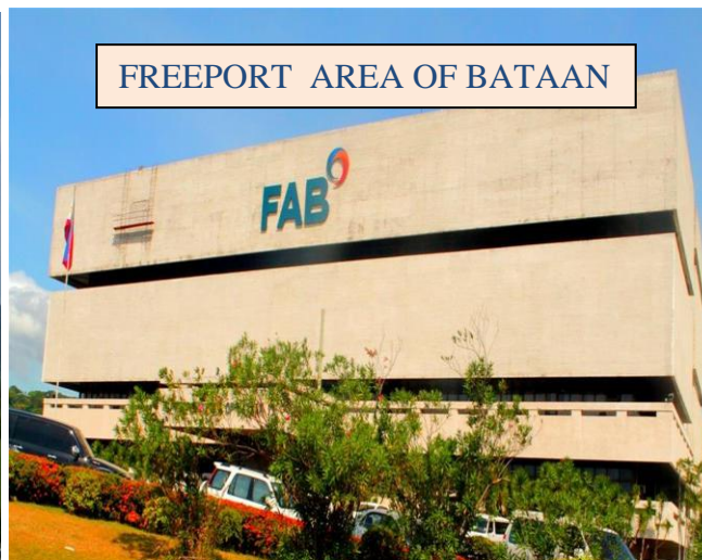
Figure 5: Freeport Area of Bataan 34 New Administration Building
